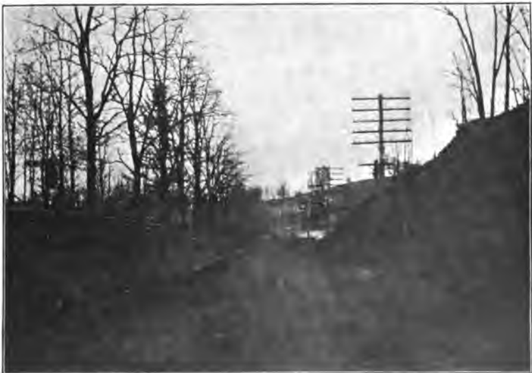
Extension Navesink road, Monmouth Co., Water Witch Club entrance, after completion.
